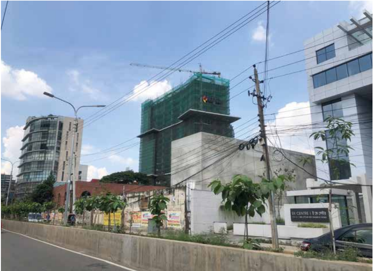
Many new constructions are taking place at both sides of the Tejgaon-Gulshan Link Road
